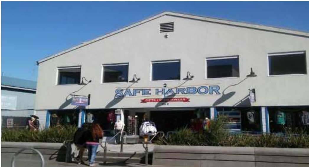
Safe Harbor San Francisco, California
